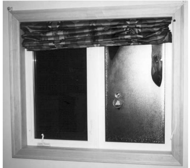
Window condensation after tight-fitting curtains are raised. The window pane on the left has low-e with argon gas fill. The fogged-up window pane on the right is conventional glass.
