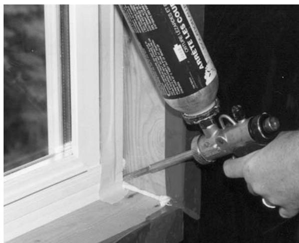
Low-expansion foam used to air-seal gap between rough opening and window frame.
